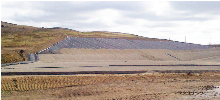
Sidewall liner keeps waste that will be disposed of in new Cell 12A from mingling with old waste in the original clay lined Cell 1 at the site.
