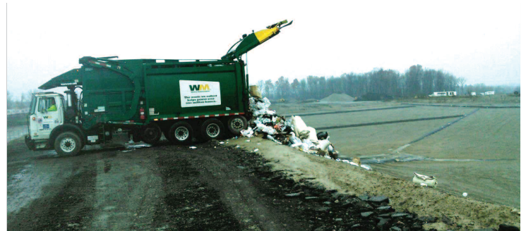
First load of waste deposited in new cell
